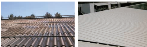
Old Roof with Sprinkler System New Roof with Insulation (40mm)
