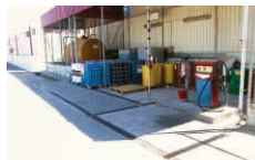
Liquids Stock Area with Gutter
