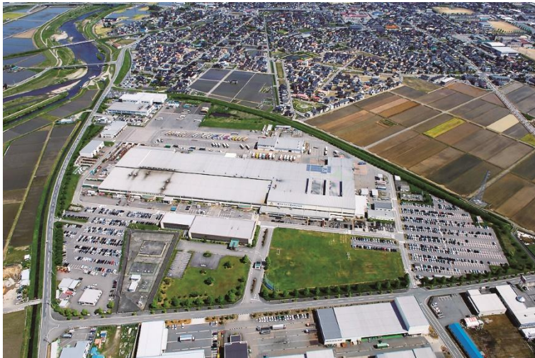
The MFBM facilities in Toyama Prefecture
